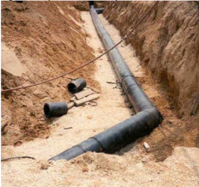
Figure 21: Pipe Placement in Open Trench
