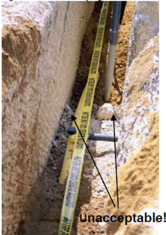
Fig. 25: Avoid Rock Impingement when Placing Embedment
