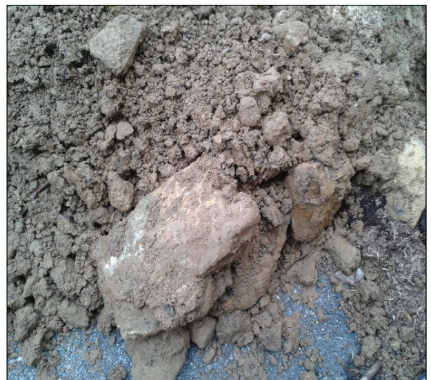
124 Springhill Road: Existing service installation with no controlled back fill and large rocks against the service line. 3
