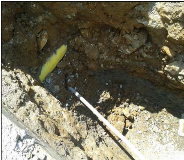
124 Springhill Road: Existing service installation with no controlled back fill and large rocks against the service line. 3
