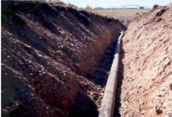
Figure 23: Trench Wall Sloped for Safety
